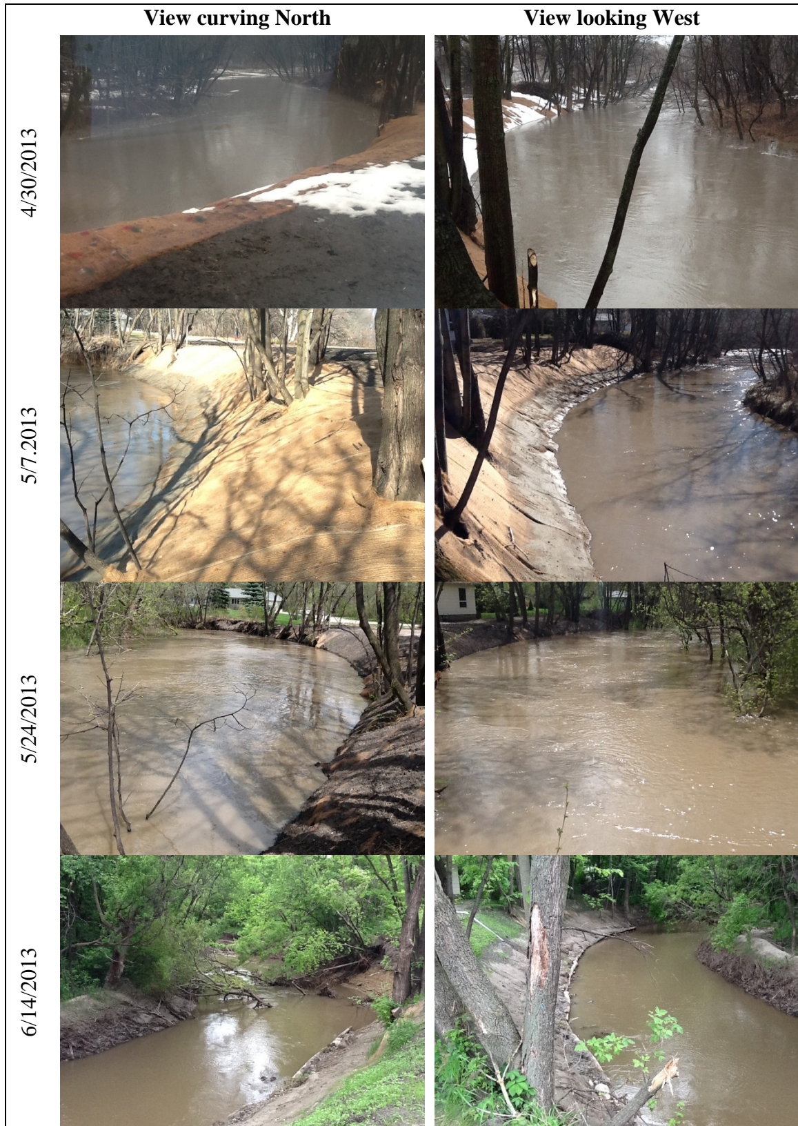
Figure 17. Photos: 2013 flooding at 201 Woodland Terrace, Cavalier, ND. Credit Neil Fedje
