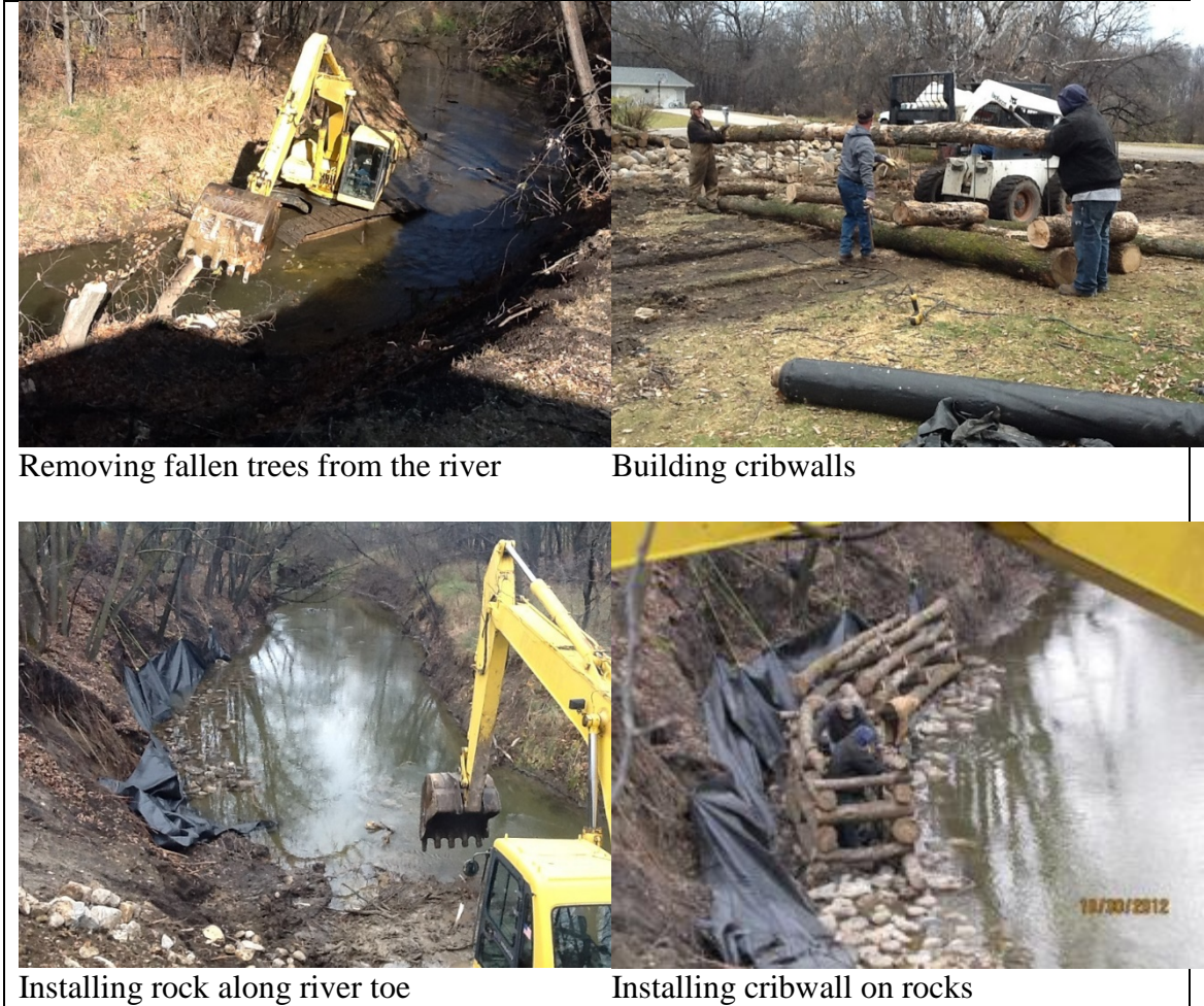
Figure 7. Photos: Cribwall installation at 201 Woodland Terrace, Cavalier, ND. Credit Neil Fedje
